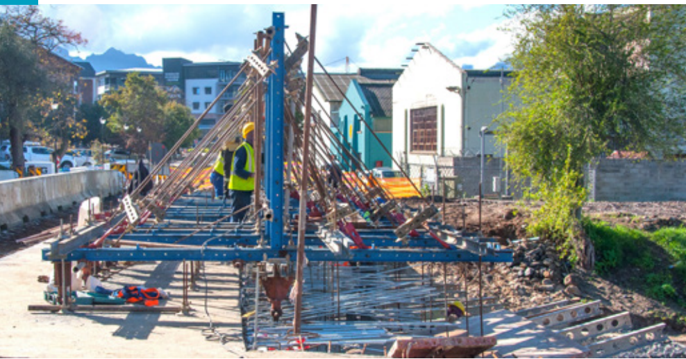
T-shaped suspension bracketing at the Phase 1 walkway mounted on pivot-point jacks
