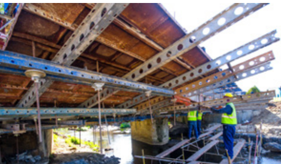
The underside girders and Econoform panelling
