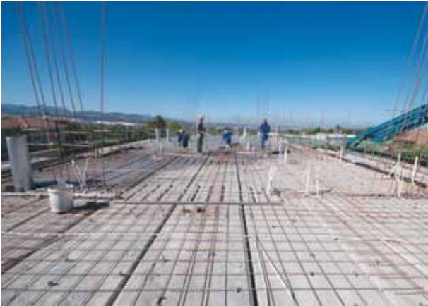
A 75mm layer of reinforced concrete is laid over a section of hollow-core slab flooring as per KLS Engineers design.
