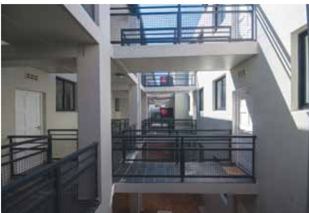
Solid-slab walkways link two of the apartment blocks.
